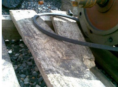
X Broken planks
