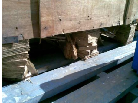
X Poor wood structure
